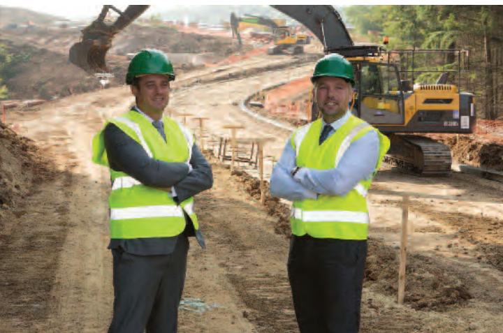
Michael Henderson, Surveying Director of Lumsden & Carroll on site in Wynyard
