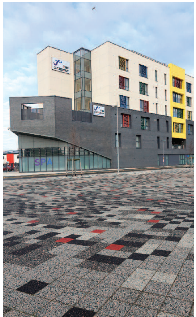
ESH BUILD: £7.2m. Design & Build. Nationally unique Neuro-Rehabilitation Centre & Transitional Housing. The Gateway, Middlehaven. RICS Project of the Year 2014 RICS - North East Renaissance Awards. North East.
