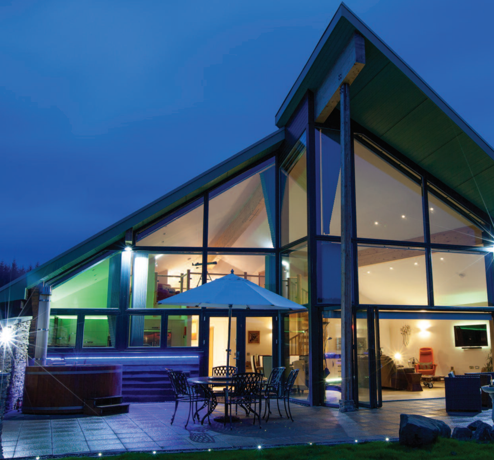
ESH PROPERTY SERVICES: £345K. Design & Build New build eco friendly holiday lodge, The Straker Lodge, Kielder, North East.
