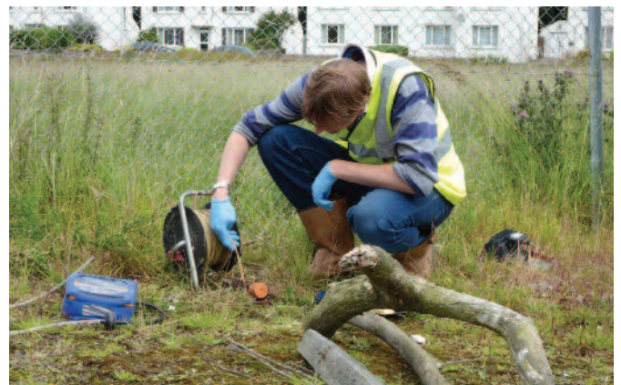
REMEDIOS: Ground remediation works, Geotechnical & contaminated land site investigation, North of England.
