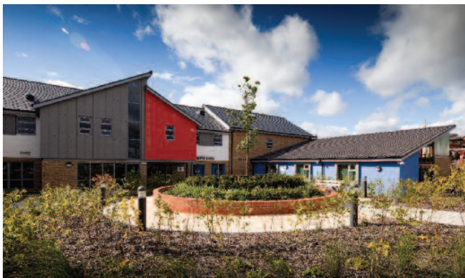
ESH BUILD: £2.9m. Design & Build. New Health Centre & Library. The Lavender Centre, Pelton, North East.
