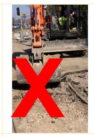
**Do not** use mechanical means of excavating **within 1m** of known services.
