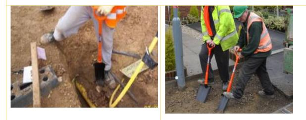
FREQUENT AND REPEATED USE SHOULD BE MADE OF CAT AND GENNY DURING THE COURSE OF THE WORK. Where services are identified add these details to your service plans including any loops, bends etc
