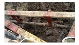
Suitable precautions should be taken to prevent damage from ongoing work in the excavation. This may involve for example the use of physical means (e.g. timber boards, sandbags etc) to prevent mechanical damage.
